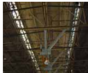
Figure 12 Application of CFRP sheet in a steel roof truss structure
