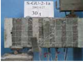
Figure 6 Debonding failure of shear strengthening using U-type GFRP
