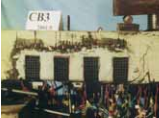
Figure 5 Debonding failure of flexural strengthening with U-type anchorage
